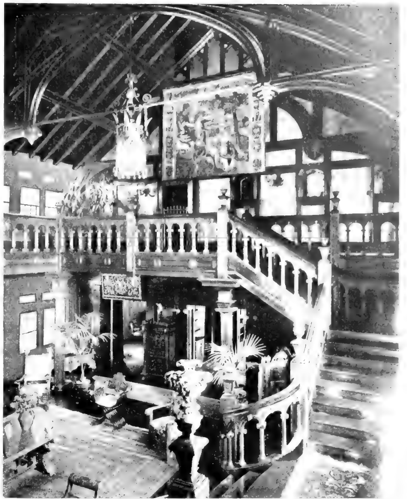
The Hall Has an Open Timber Roof
